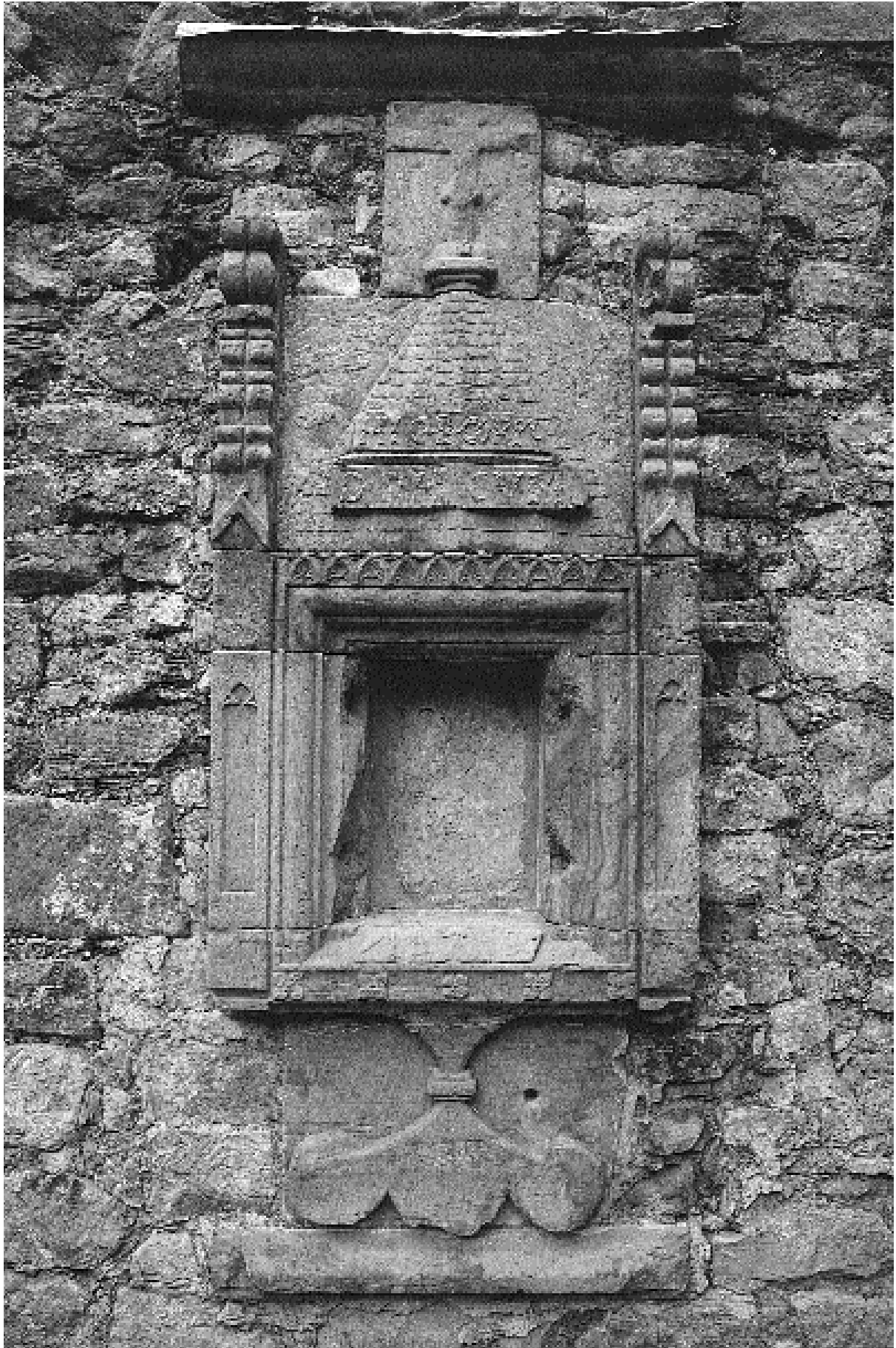
Wall Monument, Sacrament House, St Mary's Church, Auchindoir, Rhynie, Gordon
