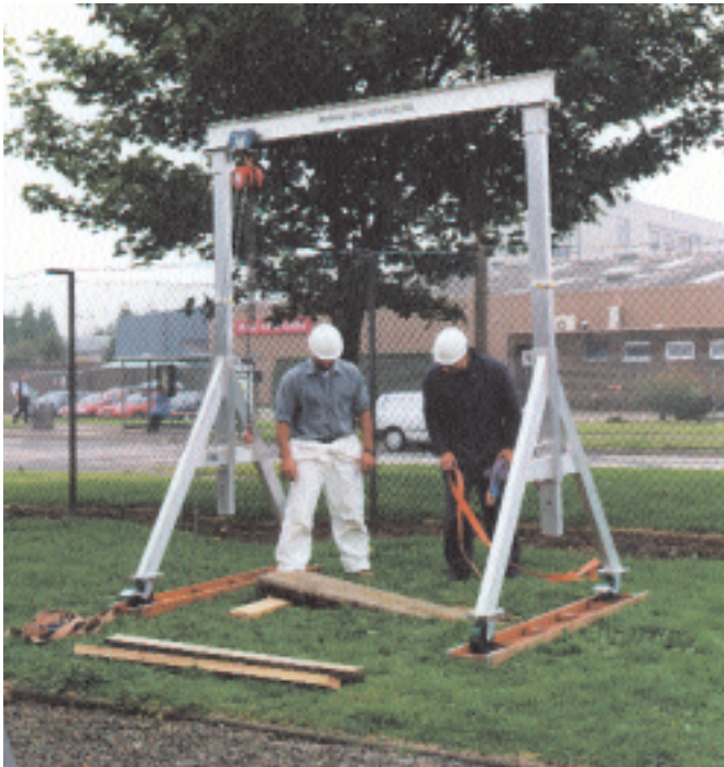
Illustration 1. Preparing to lift a stone – the A-frame is erected securely.
