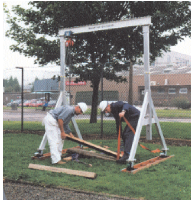
Illustration 2. Preparing to lift a stone – securing the stone to a wooden batten.
