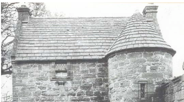
The Summer House at Edzell Castle is dated 1604 and displays a typical stone slated roof, leaded windows and oak boarded door.
